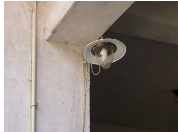
Fig. 2. Biogas light used in farmers' household corridor.
