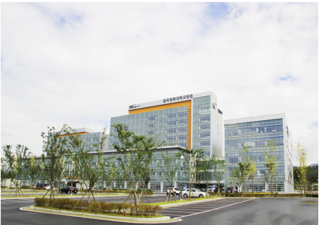
Figure 1. Exterior of the building.
