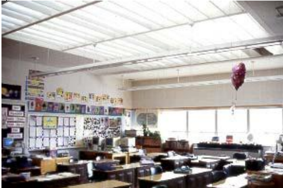
Fig. 1 - Gentle, diffuse daylight permeates a classroom with both sidelight and toplight. Note that all surfaces are painted white to distribute light more efficiently and reduce contrast glare
