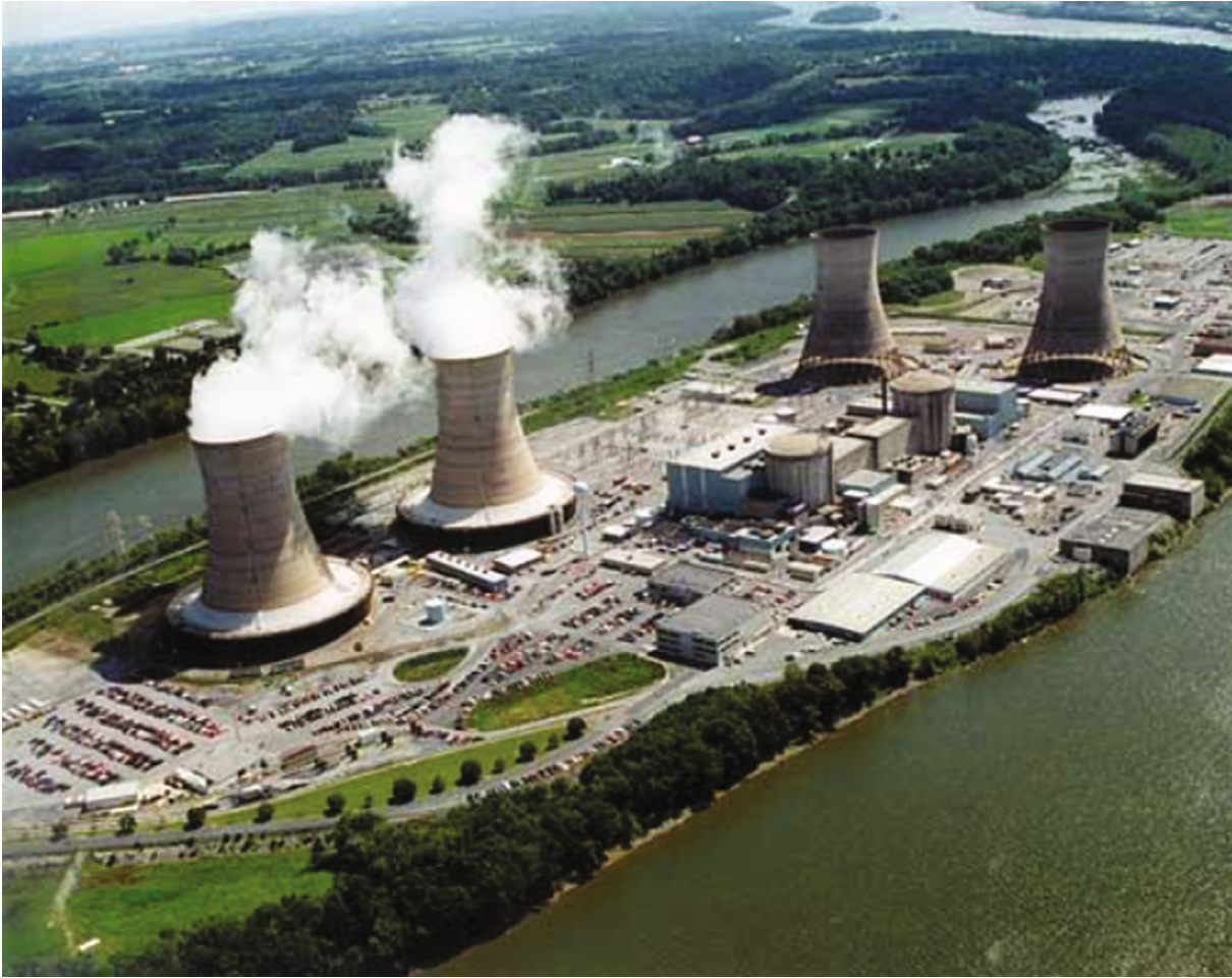
FIGURE 3: A typical appearance of a nuclear power plant (source: [16]).
