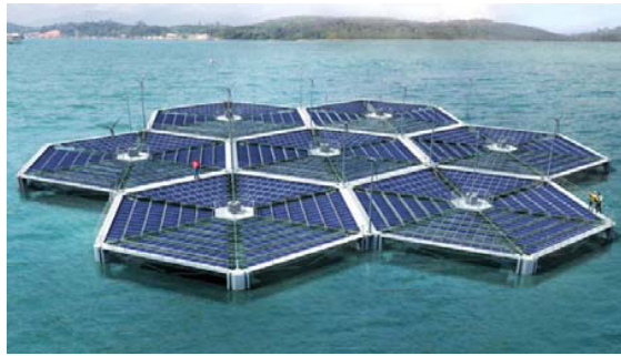
Figure 4: Power system which is combined by wave wind and solar energy generators
