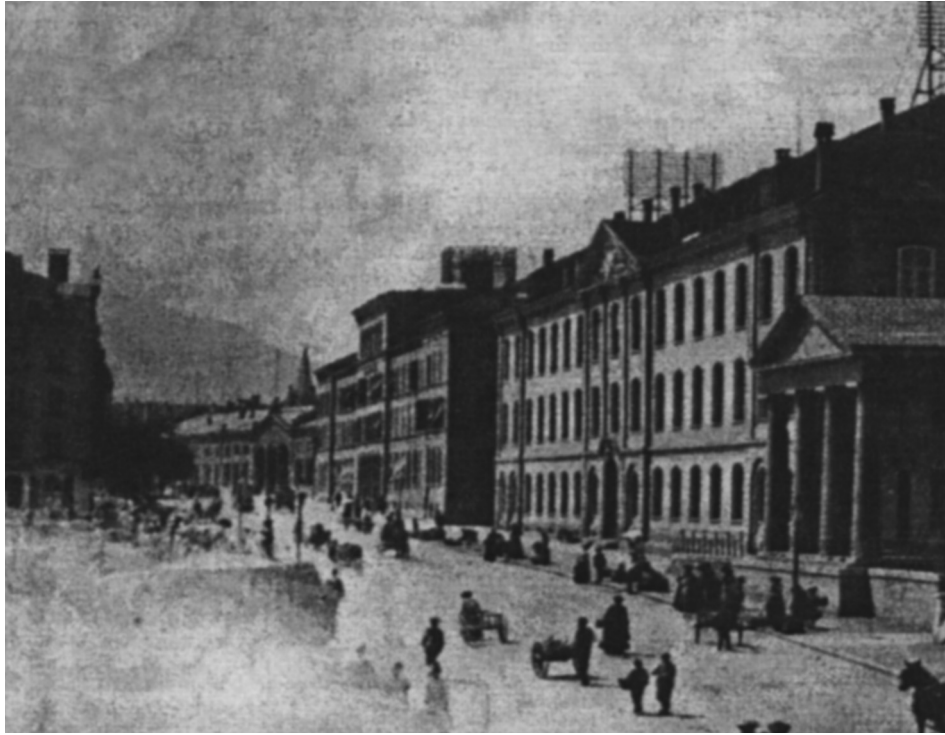
Fig. 1. The Telephone Exchange (center, directly across from the Brasserie Bollwerk at the corner of Aarberggasse) next to the Old Cavalry Barracks on Äusseres Bollwerk around 1900. The Patent Office was located there between 1907 and 1921. The three large portals of the old train station are just visible in the distance. Source: Anzeiger Region Bern , March 31, 2004, p. 1.
