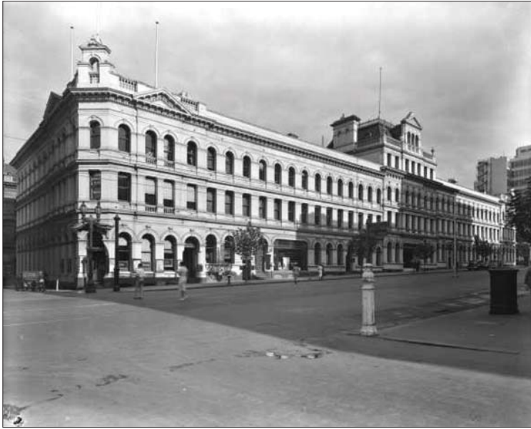
State Library of Victoria: H94.150/45 pi000295. The John Sanderson & Co wool brokers covered the entire Little Collins Street to Bourke Street block on the western side of William Street. Note the electricity supply box on the right hand side of this 1940 photograph.
