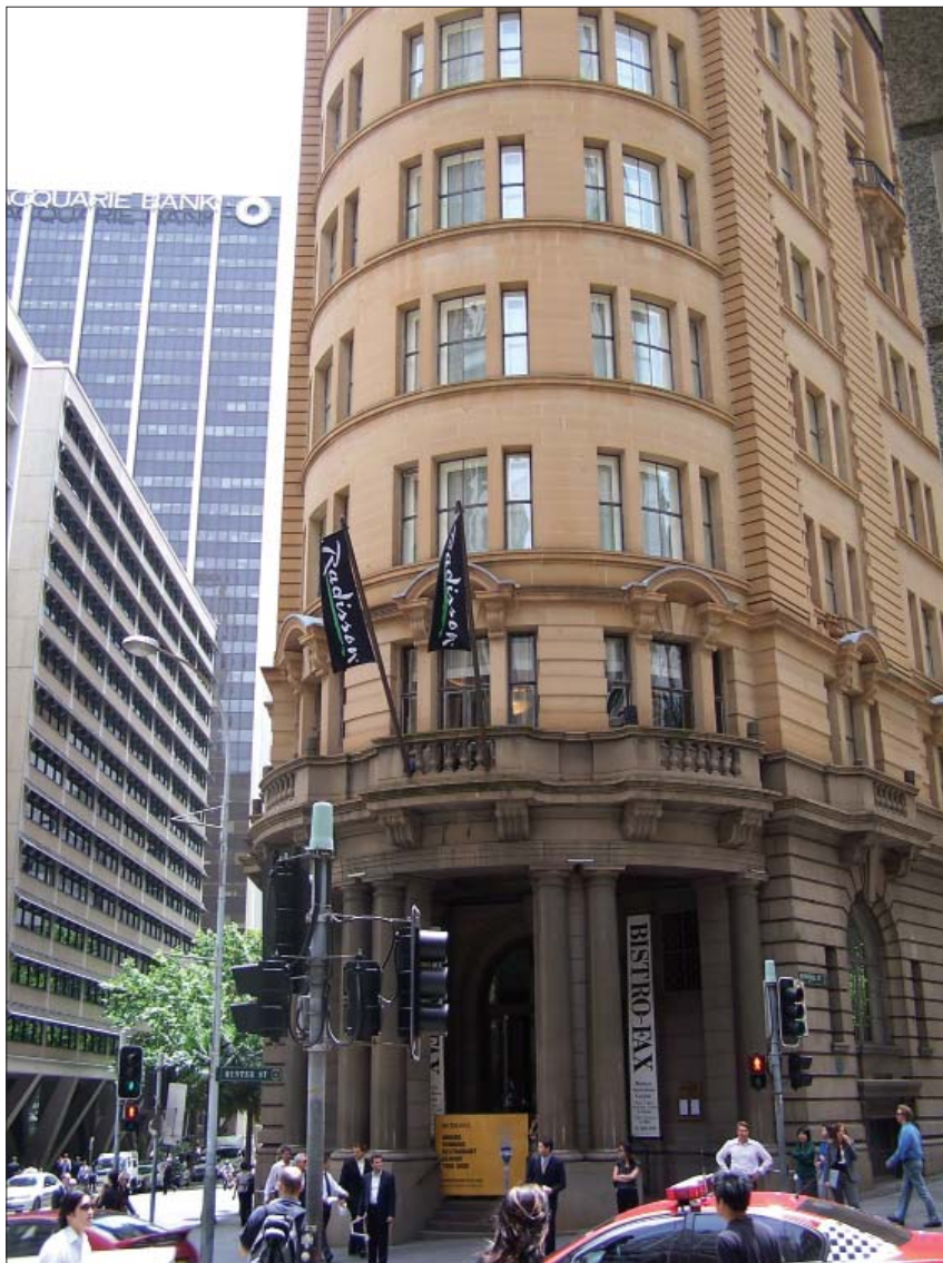
1226. The same Hunter Street, O'Connell Street intersection, with the 1924 steel framed and stone clad Herald Building on the corner.
