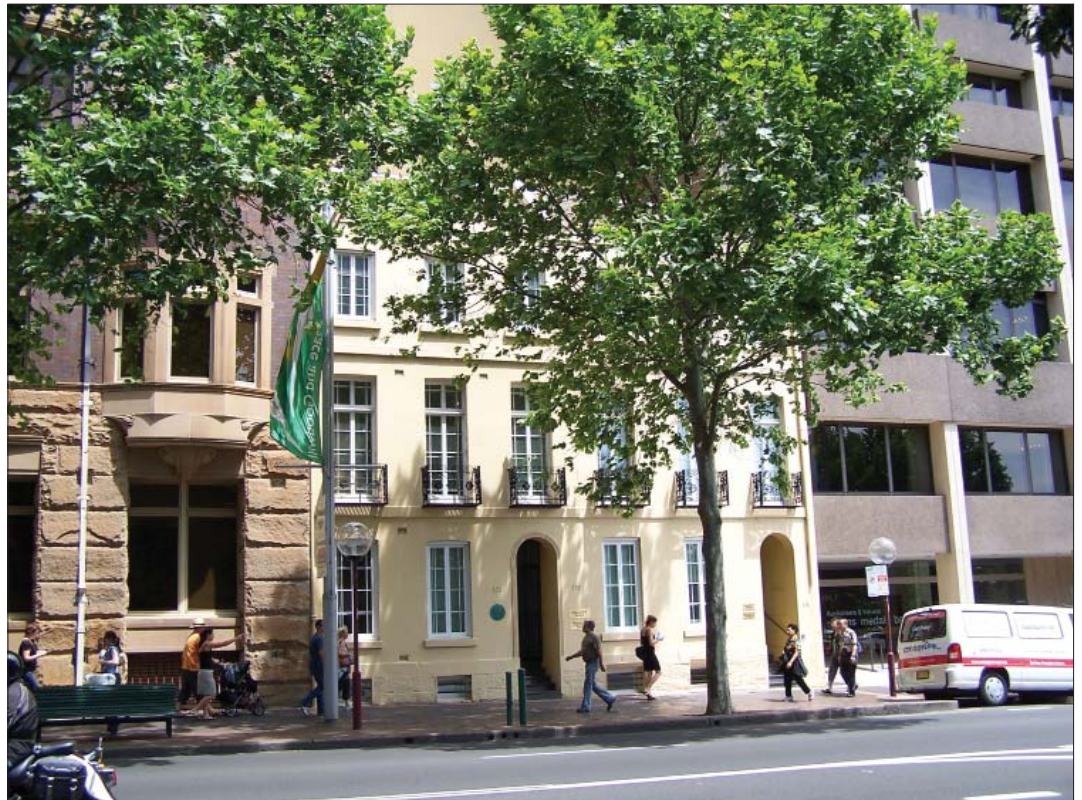
1212. Former McDonagh Medical Surgery and current Horbury Heritage Terrace at 173 Macquarie Street, now opposite the Mitchell Library. The site of the original Australia Club to the right is now just another tall city building.
