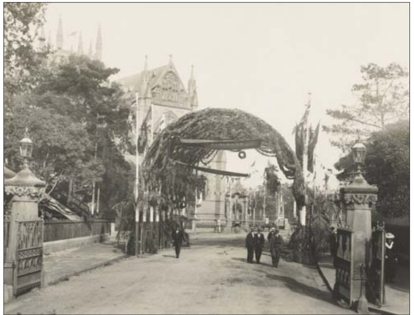
National Library of Australia: nla.pic-an 13148760-s42. The Coal Arch location looking forward through an additional floral arch to St Mary's Cathedral. This structure commemorated the visit of the Duke and Duchess of Cornwall and York late in May 1901, on their return from the opening of the Federal Parliament in Melbourne. A century ago, there were fewer trees, and the road surface is indicative of horse transport rather than the later automobile.
