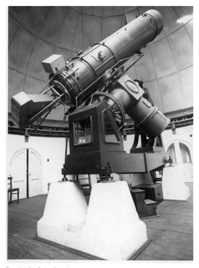
Figure 20.4: Zeiss-Gautier reflector telescope
