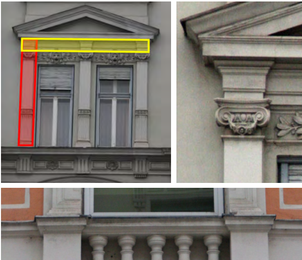
Figure 11: Examples of a window with overlapping structures. The pilaster (red) overlaps the architrave (yellow). In the overlapping area, the moulding of the architrave runs across a continuation of the capital of the pilaster. In the window at the bottom, a ledge that runs across the whole façade also serves the purpose of a window sill.
