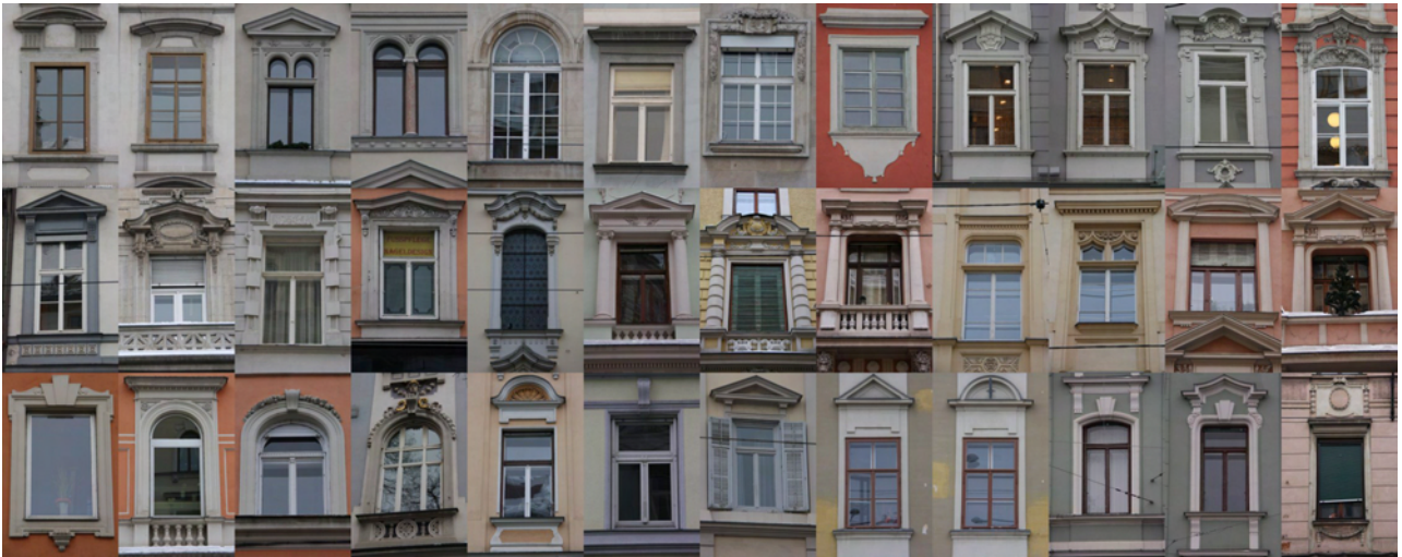
Figure 2: Window exemplars. The full set contains 150 images of windows from neo-classical buildings erected in Graz, Austria, in 1860-1890 ( Gründerzeit ). The complexity and visual dominance of the windows pose challenges to any digital urban reconstruction.
