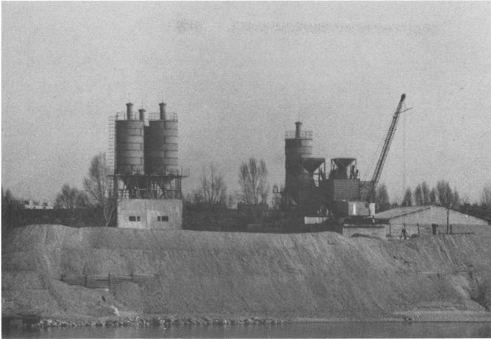
Fig. 9(a). Building construction machinery on the bank of the Danube.
