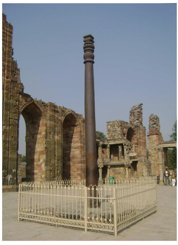
Figure 4.1: The famed rust-less iron pillar installed in Delhi in about 1233 CE was originally erected as a gnomon in Udaigiri, central India, located on tropic of Cancer. The gnomon, built about 400 CE was designed to cast shadow in the direction of the passage to temples, on summer solstice day. (Photo courtesy R. Balasubramaniam)
