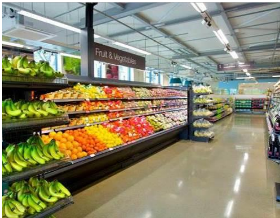
Figure 3 Lower ambient light levels leading to lower energy consumption (source: Philips Lighting)
