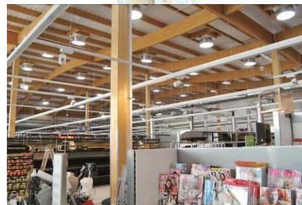
Figure 9 Daylight guidance systems using light-pipes (source: Monodraught).
