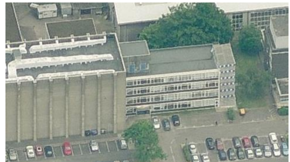
Figure 14 Glazed façade office building proposed to be lit by a net zero energy lighting system
