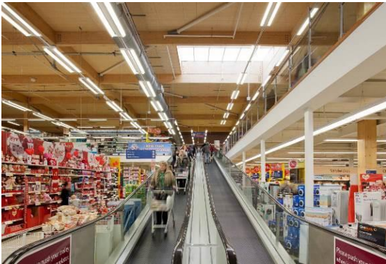
Figure 11 Daylight-based, dimmable T5 fluorescent fittings with adjustable reflectors and louvres producing the right light output at the level of the merchandise (source: Whitecroft Lighting)
