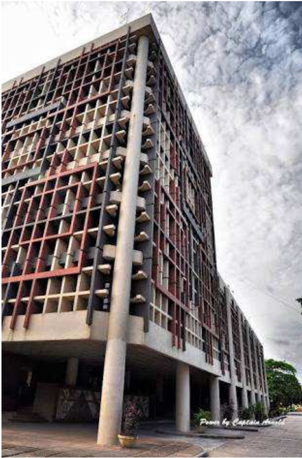
Figure 4. Note the platform, column arrangement and effect of the facade on building texture [9].
