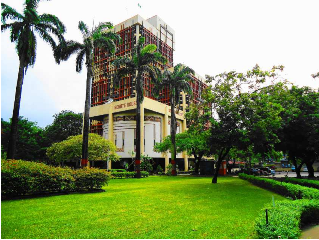
Figure 6. The earth toned colors add an ethnic feel to the building's aura [11].
