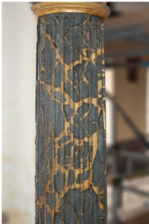
FIGURE 3 The grand columns in St. George's Chapel, Great Yarmouth, England (1714), painted using smalt and gold to simulate lapis lazuli.
