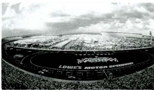
Aerial view of Lowe's Motor Speedway, considered the hub of NASCAR in the Southeast.
