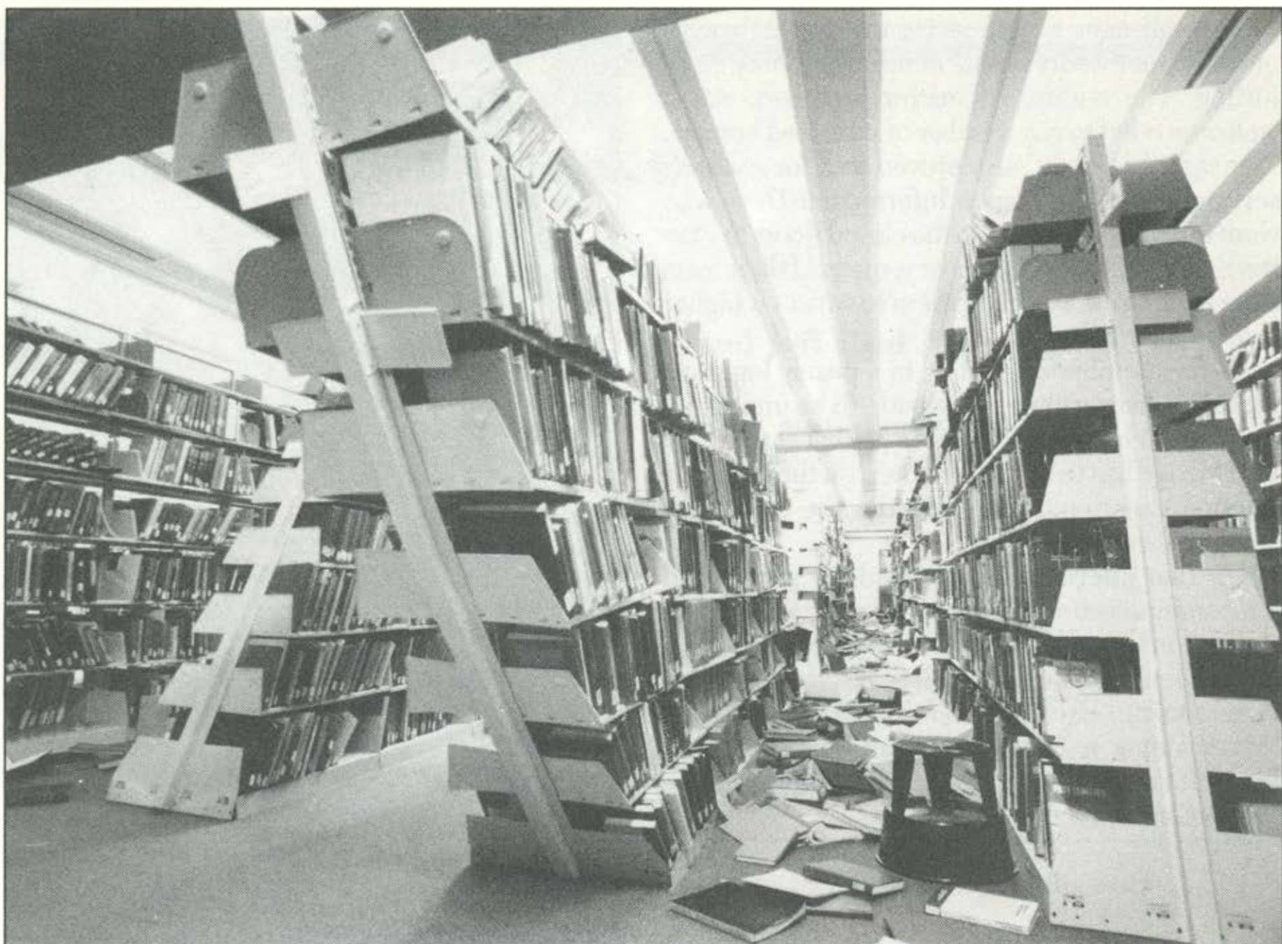
More damage to upper floors of Clark Library, San Jose State University.
