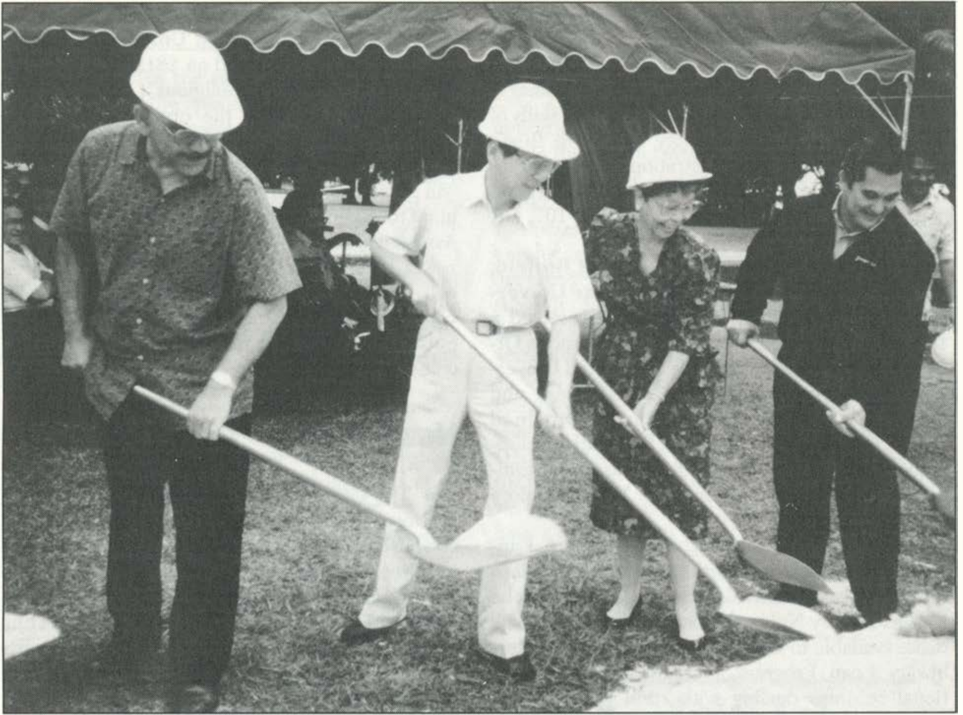
Groundbreaking ceremony at the University of Guam, Mangilao.
