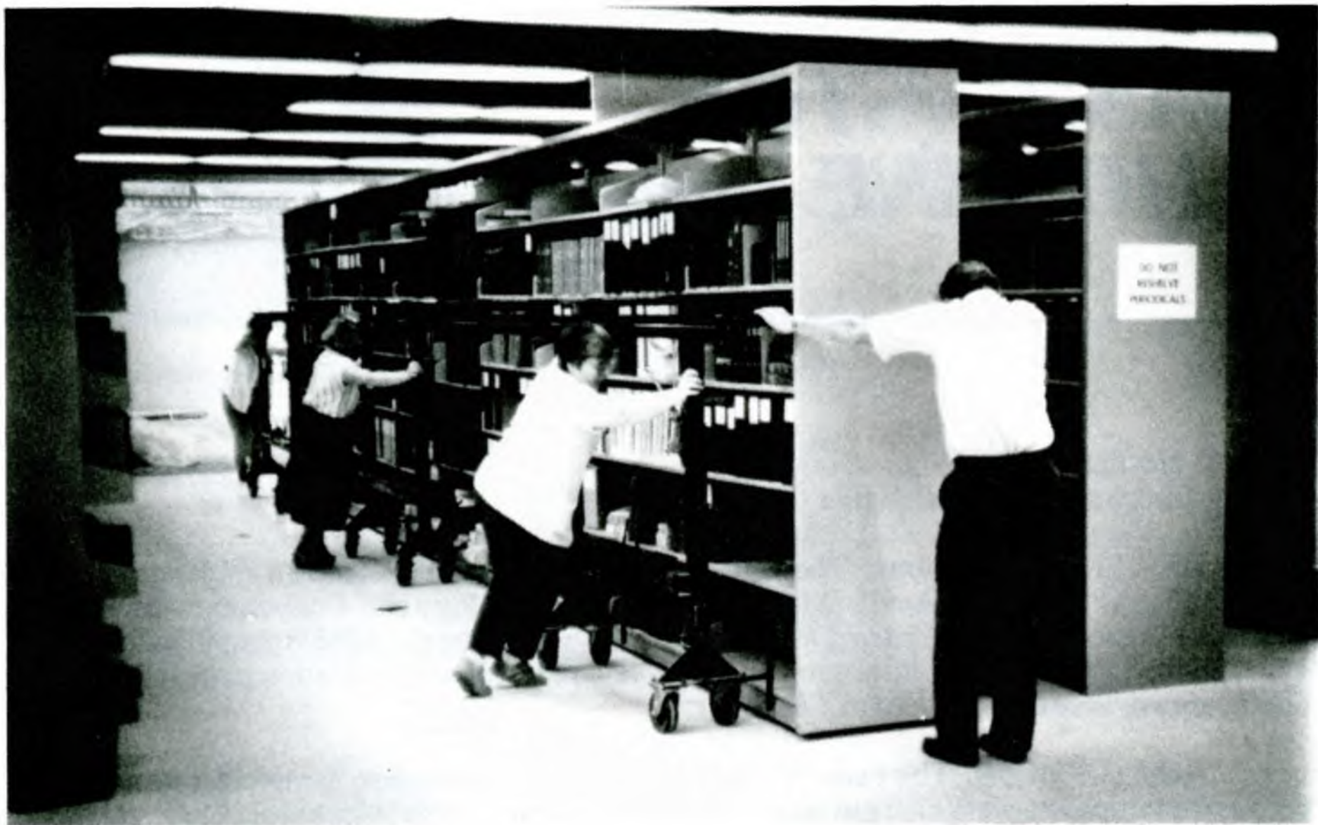
The stack-mover allows for easy shifting of stack ranges.
