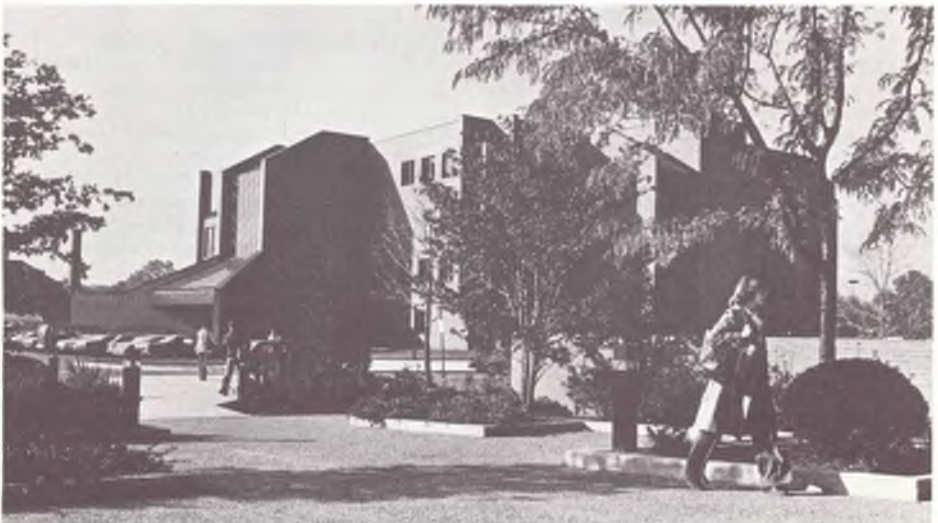
Northeastern Illinois University's new library building is among the largest building projects of the university's history.
