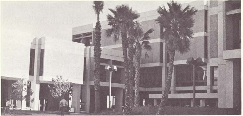
Univ. of Arizona Library exterior (above) and interior (below).
