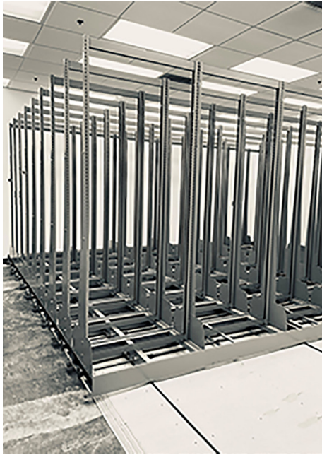
The Poetry Center's compact shelving project midway through installation. Photo by Sarah Kortemeier.
