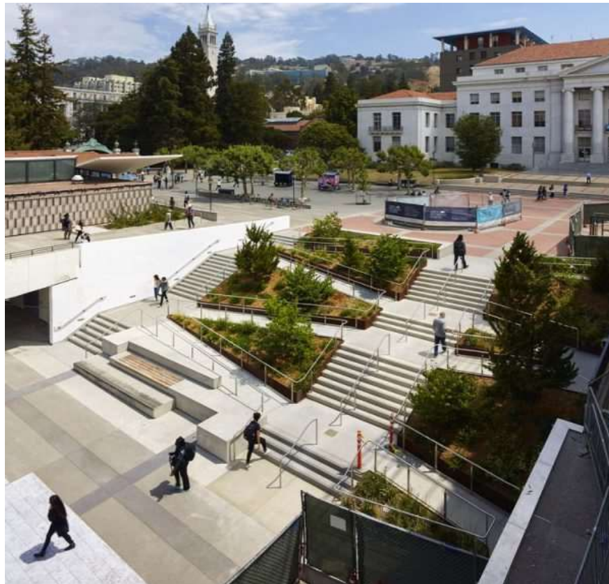
Fig. 6 (a) An inclusive landscape design of the front of a public building complex, with the disabled wheel chair users (as below) in mind (source:.. Dunlop & Hawking, 2019).
