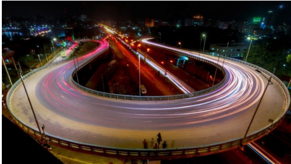
Figure 5: U-loop near Rampura TV Station
