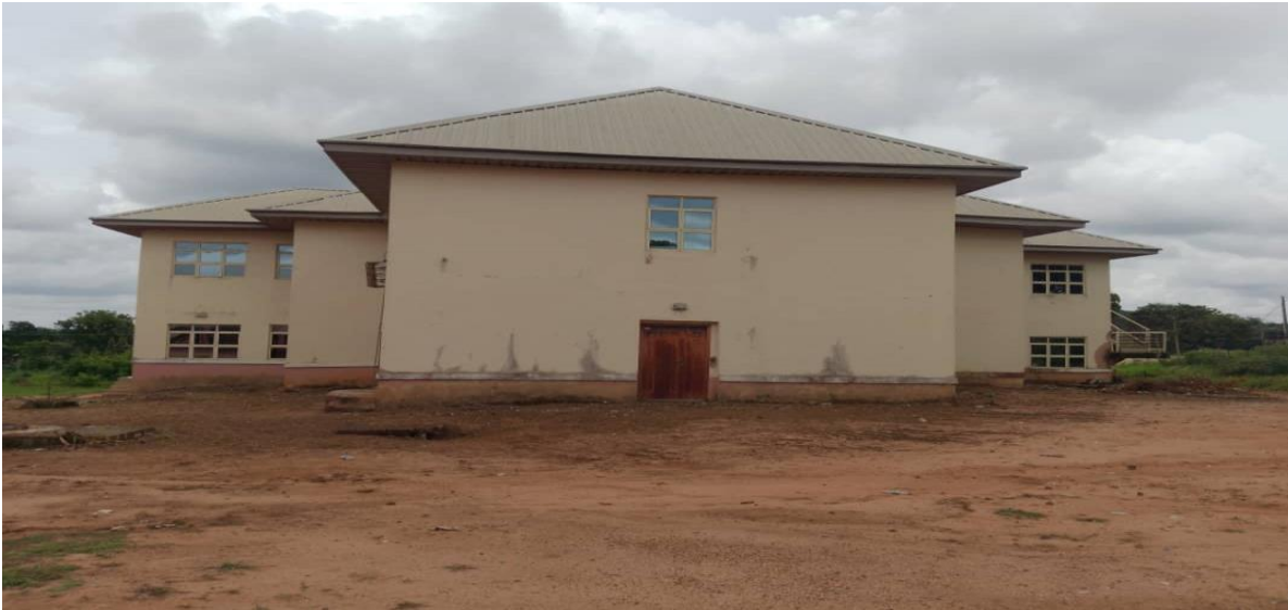
Figure 19 Rear View as built
