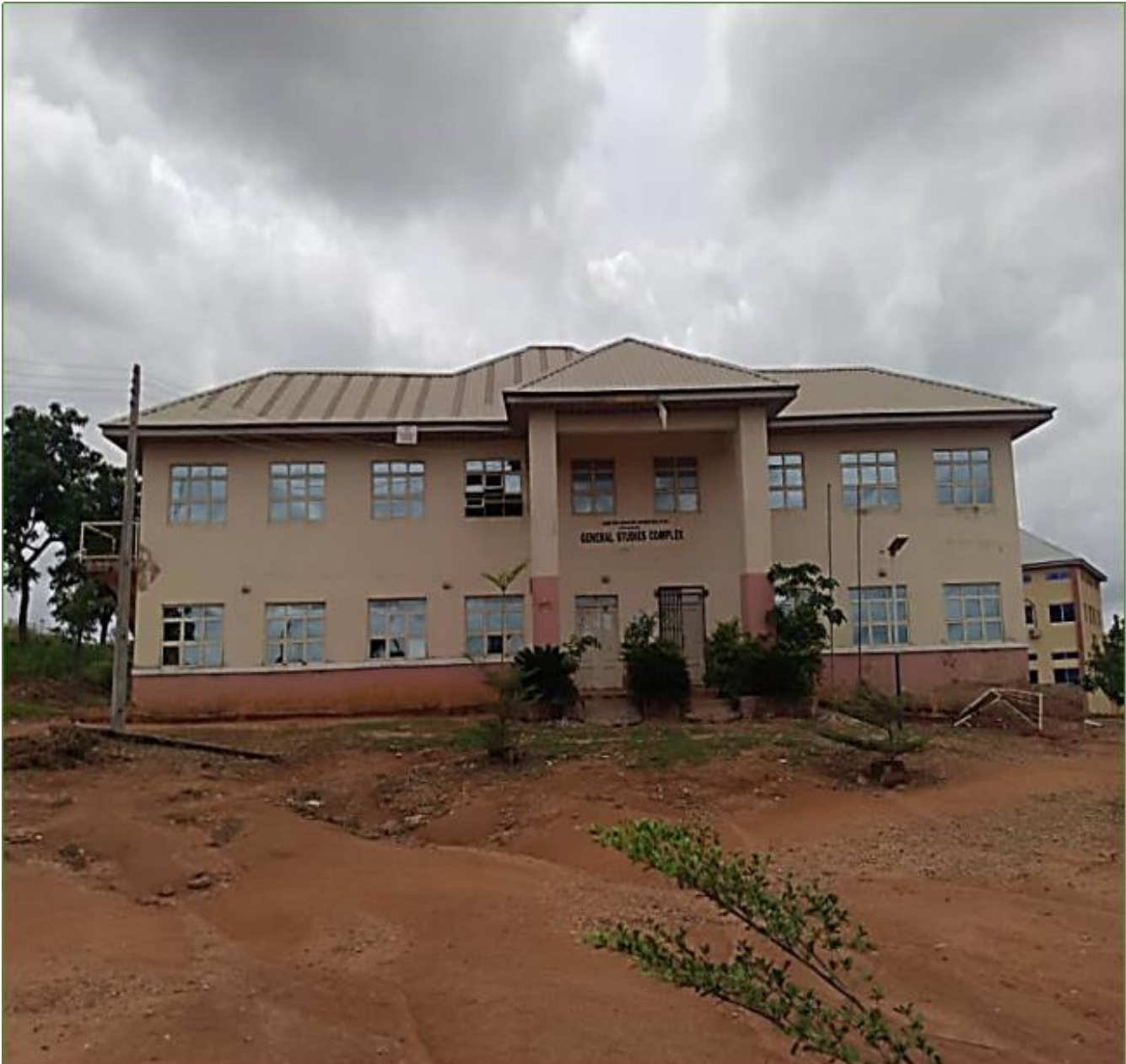
Figure 18 Approach View as built
