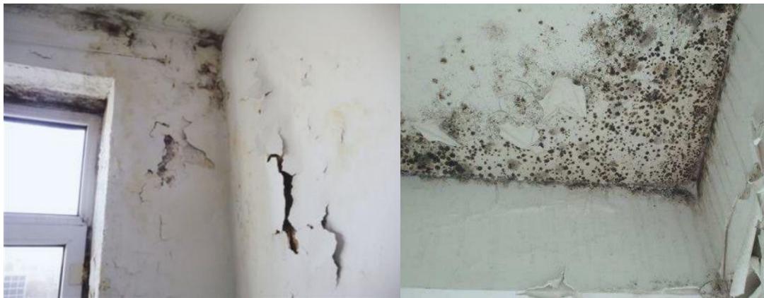
Figure 4. Current Situation of Internal Walls
