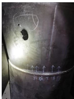
Figure 12. Wall wear and perforation of cyclone separator
