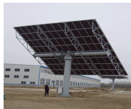
Figure 1. Schematic diagram of heliostat and base ( https://baike.baidu.com/item/%E5%AE%9A%E6%97%A5%E9%95%9C/9109957 )
