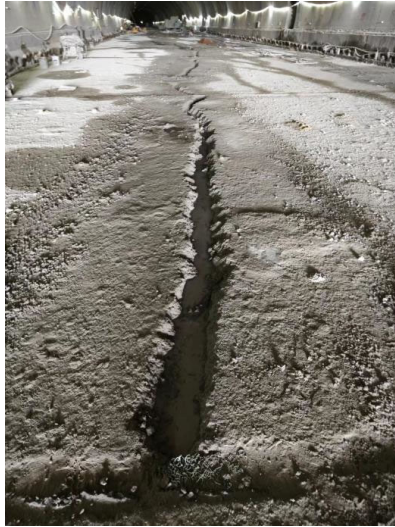
Figure 2. Through-crack slotting diagram
