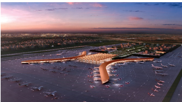
Fig 1. Cambodia Phnom Penh Tak Chong Airport Project Overall Effect
