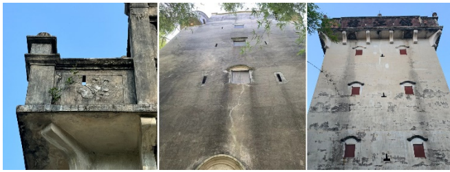
Figure 7. Firing Holes on the Exterior Walls of Kaiping Diaolou.
