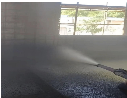
Figure 2.2. Test injection process 2
