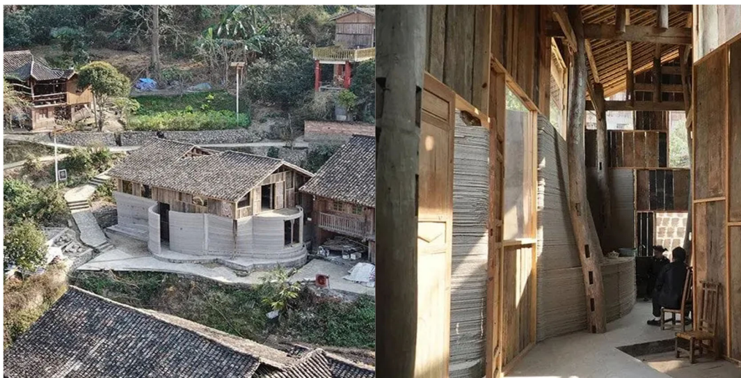
Figure 8. The integration of wooden architecture and 3D-printed concrete in Nanlong Village
