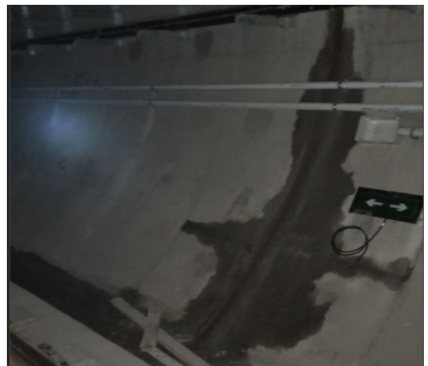
Figure 10. Joint leakage
