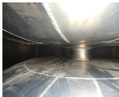
Figure 2. Inside of Closed Space Simulator
