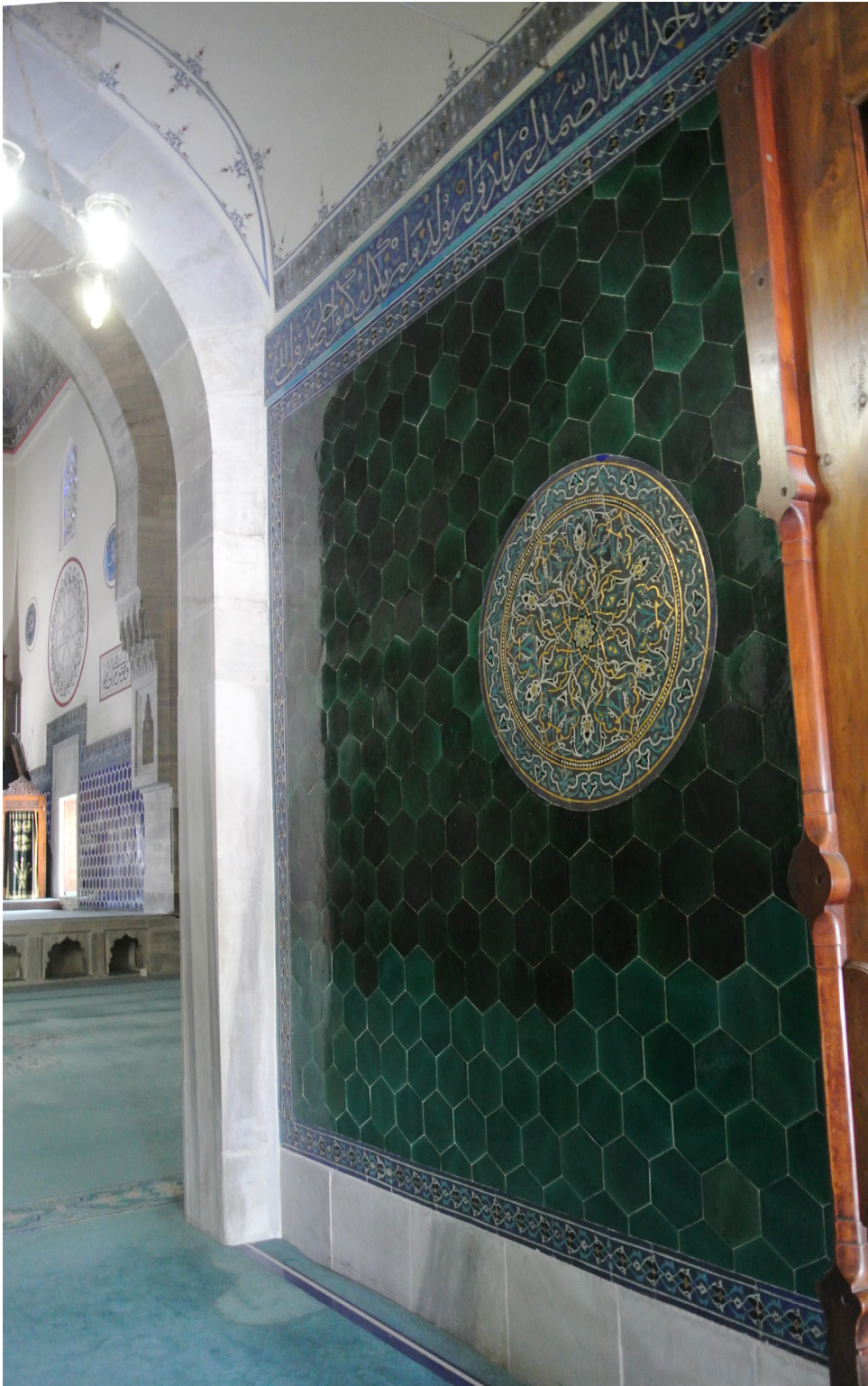
Fig. 15. Monochrome tile with black-line tile medallion in the hallway between vestibule and prayer hall, Mehmed I's mosque-zāviye, Bursa, 1419–21. Photograph by the author, 2016.
