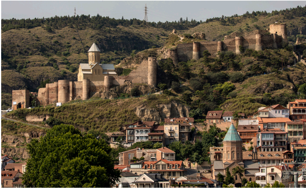
Fig. 7. The heavily restored Kala Fortress above T'bilisi's old city. Photograph by the author.
