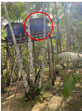
(C). Main tank.
