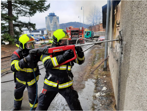
FIGURE 2. Firefighters using COBRA equipment [7].
