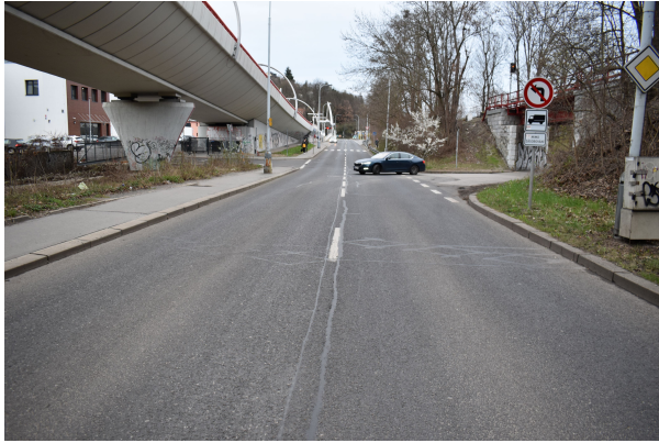
FIGURE 1. Induction loops on Hlubočepská street.
