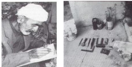
Figure 11: This image dates to the early 1970s when construction was carried out by one of the most famous builders in the city of Hebron, Rabieh Abu Hikal with his tools (source Hirschfeld, Yizhar.1995)
