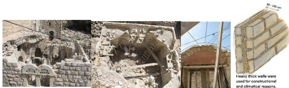
Figure 3: Image of construction material used in building a traditional. (Rehabilitation comity in Hebron, 2020) (Drawing by Author 2023)
