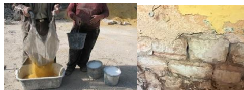
Figure 16: Shows the final shape of the vault after the decoding of the bricks (rehabilitation comity in Hebron 2020)
