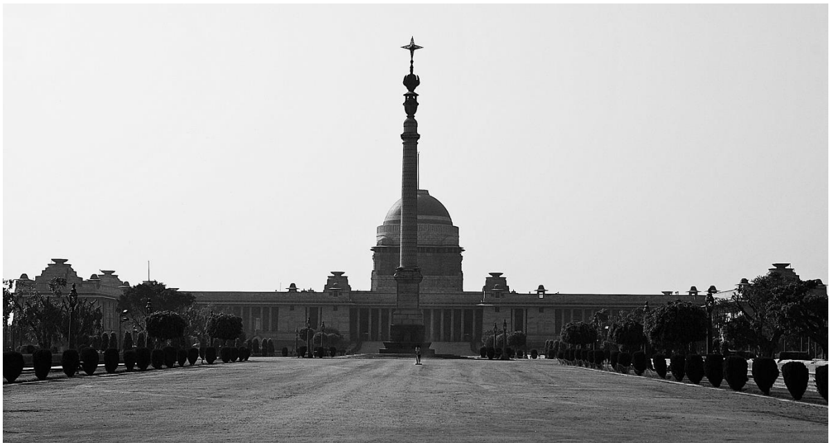
Figure 7: Viceroy's Residence / Rashtrapati Bhavan. Note the individual sweeping the grounds in the foreground, easy to overlook in the context of the monument in the background. The bottom floors of the Viceroy's Residence which support the range of functions mentioned prior, are comparably easy to overlook, buried in the proverbial "plinth" upon which the more-visible architectural language rests. (Source: Adaptorplug, 2009)
