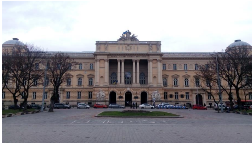
Figure 7: The Building of the Galician Sejm in Lviv, 1877-1881, arch. J. Hochberger (Source: by the author)
