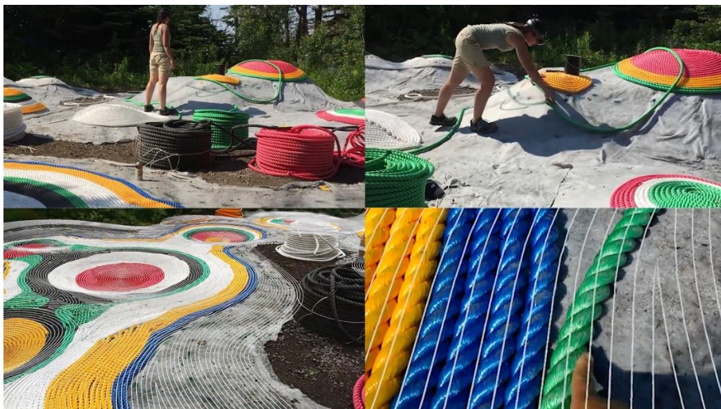
Figure 8: Images illustrating the in-situ fabrication process of Augmented Grounds .
