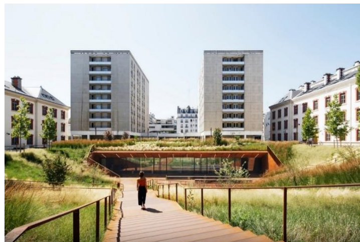
Figure 22: The location of the project within old military barracks (University of Law Paris I, Paris 13 - ChartierDalix, n.d.)
