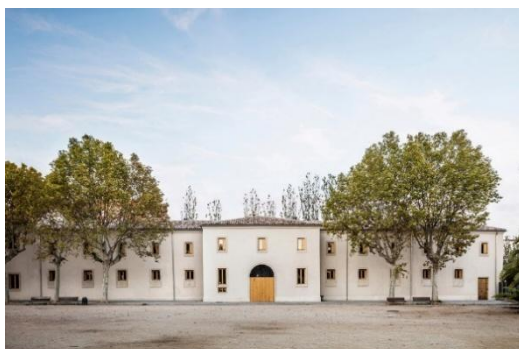
Figure 14: Exterior view of building after renovation (Villa, 2019).
