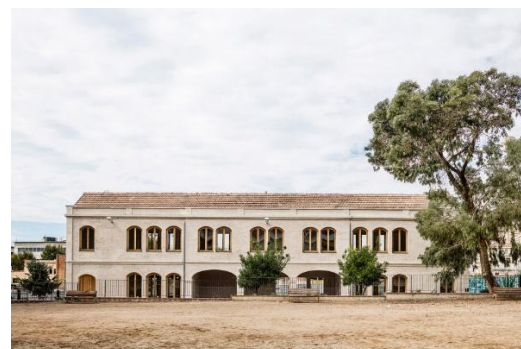
Figure 15: Exterior view of building after renovation (Villa, 2019).
