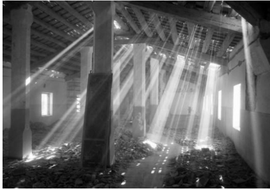
Figure 16: Before restoration (Villa, 2019).
