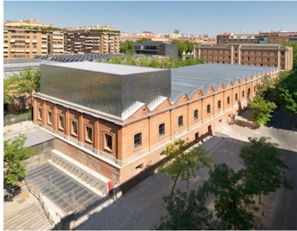
Figure 7: Roof Sawtooth (Valenzuela, 2024).
