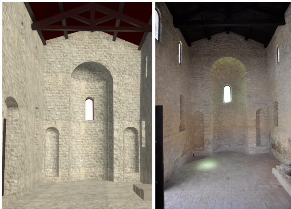
Figure 2: Internal views of the San Giovannello. Form left to right: a view of the model (Autodesk Revit) and a photograph of the inside of the church (Graphic elaboration by Serena Buglisi).
