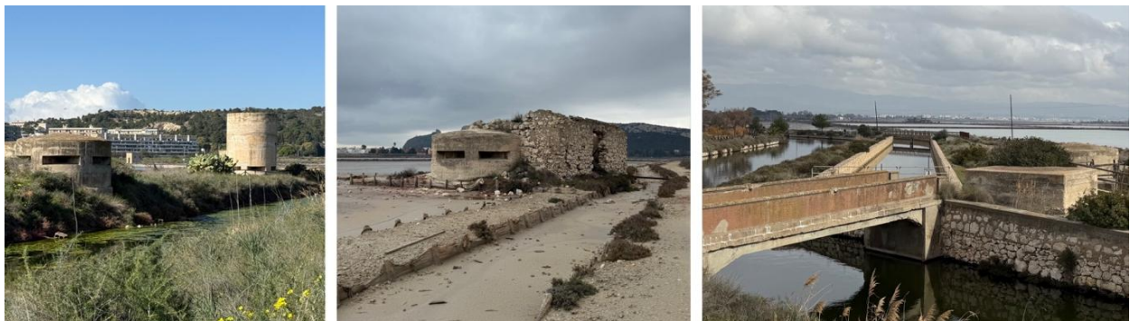
Figure 17: From left to right, stronghold No. 15, a double casemate bunker belonging to the Stronghold No. 16, and two bunkers belonging to the stronghold in Sardinia, Italy (photos by G. Sanna-author, 2025).
