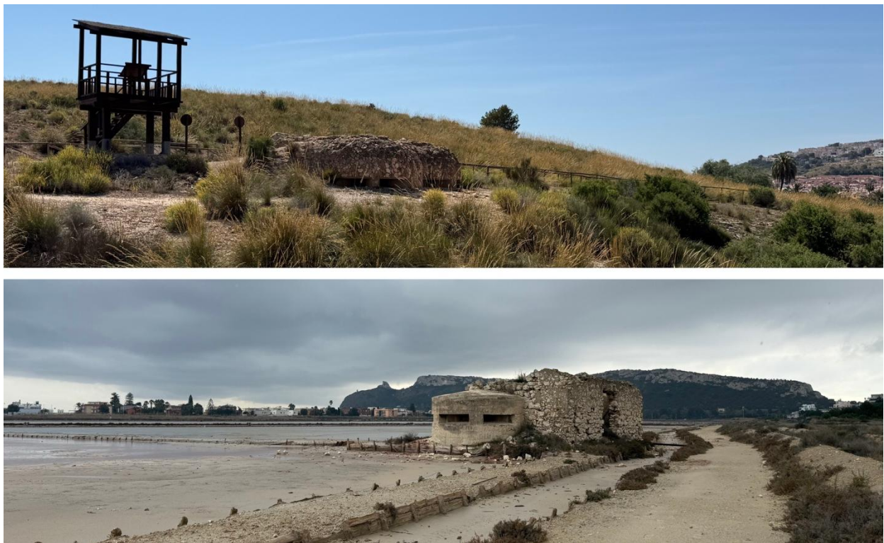
Figure 18: Comparative views of two double pillbox bunkers: Clot de Galvany in Spain (above) and Molentargius in Italy (below). (photos by G. Sanna, 2025-author).
