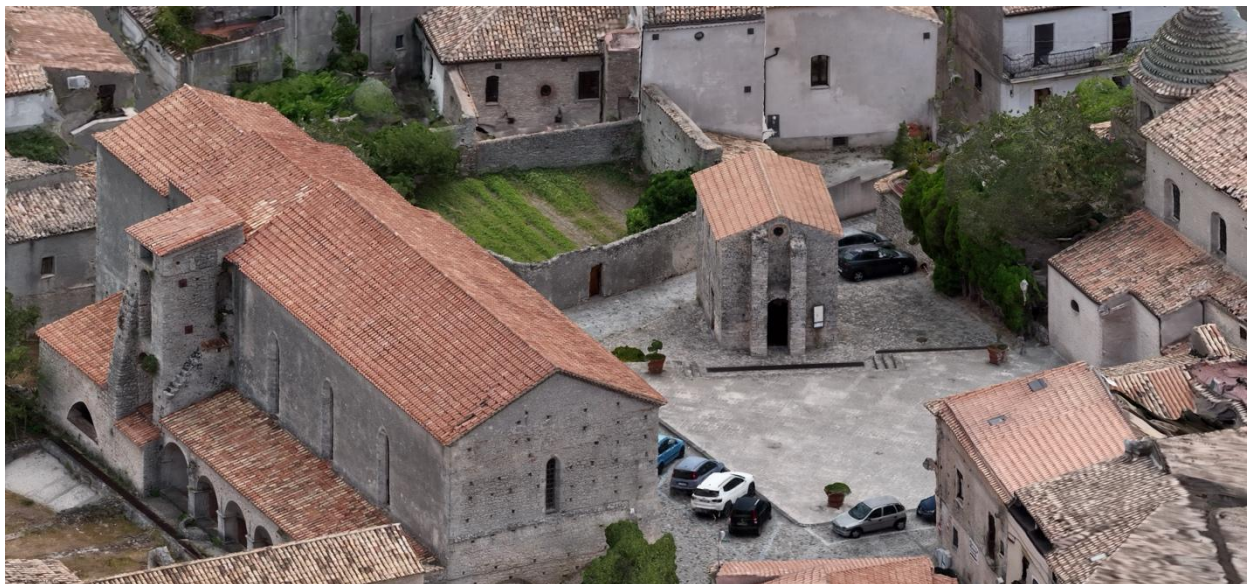
Figure 4: The convent and the church of S. Francesco (left), the church of S. Giovannello (center). View of the textured mesh obtained by the union of different survey techniques (terrestrial photogrammetry, aerial photogrammetry, laser scanner). (Graphic elaboration by L. Pizzonia.)
