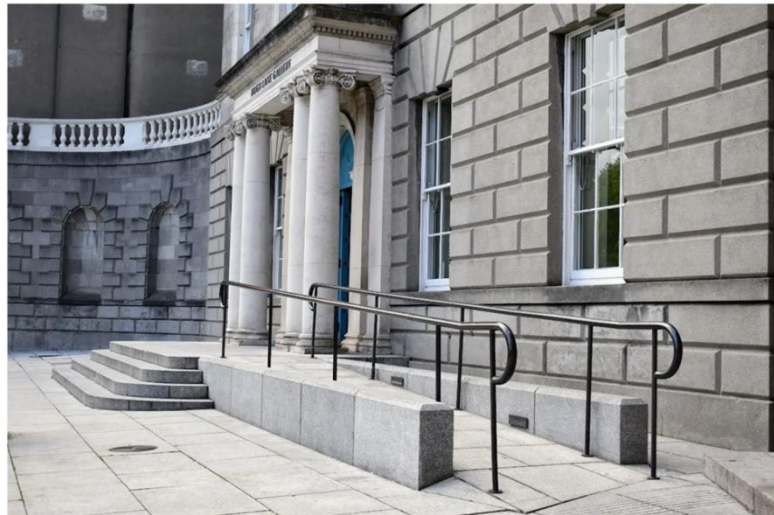
Figure 1 – Adding a ramp to make the entrance accessible. The Hugh Lane Gallery (Source: https://hughlane.ie/accessibility-2/ )
