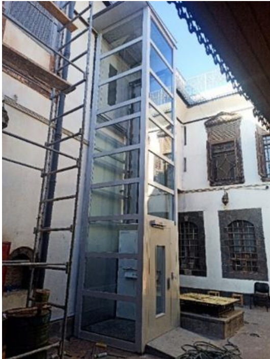
Figure 5. (a) – Added elevator with a contemporary design. Fakhri Al-Baroudi House
