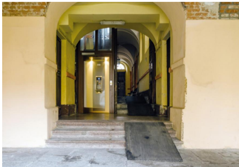
Figure 2 – Architectural intervention to add a lifting platform with a temporary ramp. The Collegio Cairoli (Elevatori Magazine, n.d.)
