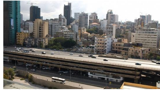
Figure 8: Viaduct Charles Helou Source: mascontext.com
