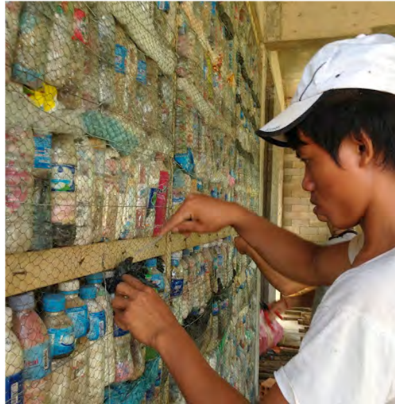
Figure 7. A youth working on building vertical plastic bottles wall in Cambodia. [14]
