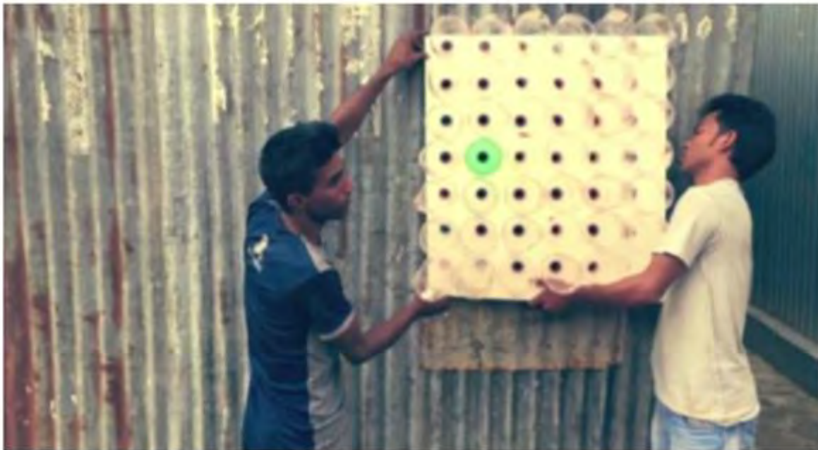
Figure 6. Two men installing a zero electricity air conditioner [13]
